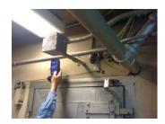
The meter nulled when held right under this conduit. There had to be two conduits in order to cause the problem and they ended up being about 8ft apart.
